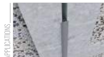
50 mm gap for stainless steel corner
